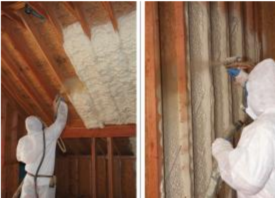
Gambar 28 Metoda semprot untuk aplikasi material insulasi termal. Sumber: http://www.greenbuildingadvisor.com/blogs/dept/green-building-blog/procon-open-cell-or-closed-cell-foam
