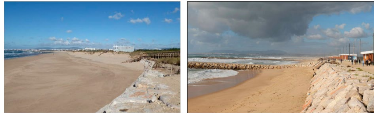
Pembangunan coastal barriers ( hard engineering ) yang memanfaatkan artificial sand nourishment ( soft engineering ) di Costa da Caparica
