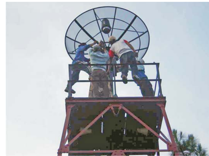
Gambar 14: Instalasi Small Radio Telescope 2.3 m di Observatorium Bosscha (sumber: Dr. Taufiq Hidayat, Observatorium Bosscha)
